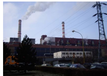
The TEKO station for heat production
