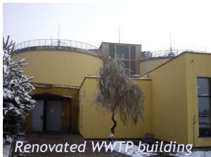
Renovated WWTP building
